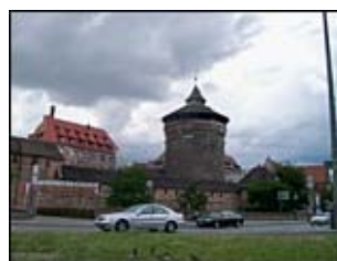
Roman water tower left near original gate into Nuremberg
